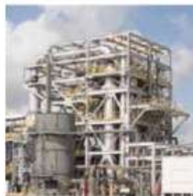
Step 3: Gas clean up and syngas heat recovery
