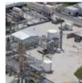
Step 6: Renewable power generation
